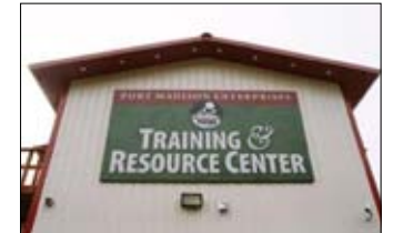
Suquamish Tribe's Port Madison Enterprises is one of the largest employers in Kitsap County with more than 780 employees. The new Training and Resource Center is being housed in an existing building that was acquired and is being remodeled and improved.
